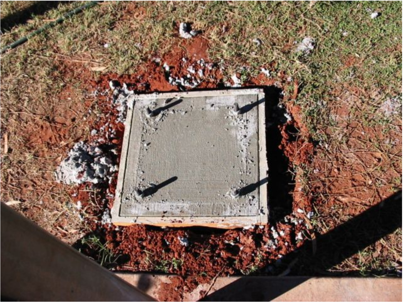
THE CONCRETE PAD. ABOUT 350mm SHOWN, BUT IT'S 500mm X 500mm SQUARE AND 850mm DEEP.
